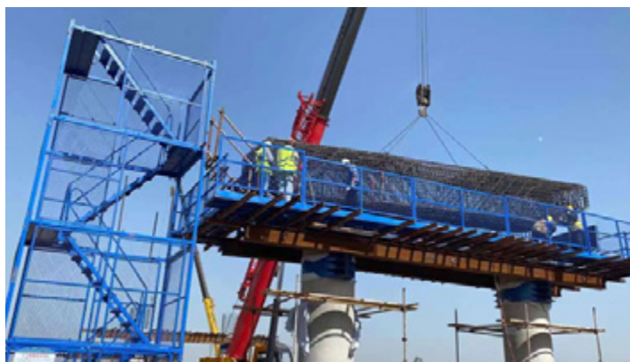
Steel Formwork for Bent Cap 盖梁钢模板
