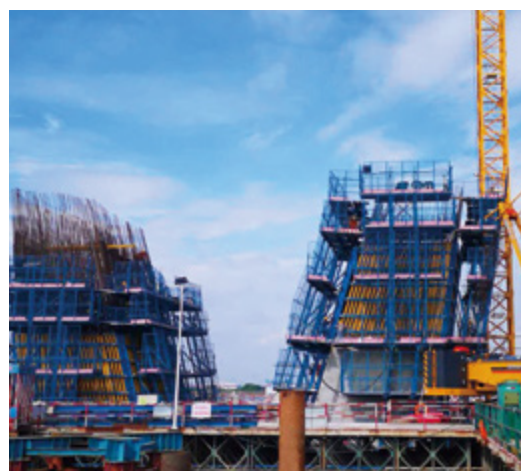
Climbing Formwork for Pier 墩柱爬模
