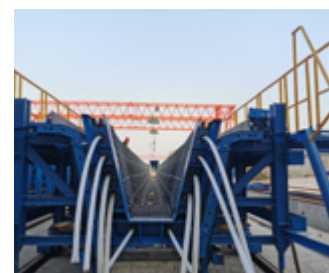
Prefabricated Box Girder (Hydraulic) 预制箱梁 ( 液压 )
