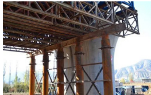
Beret Beam Support 贝雷梁支架
