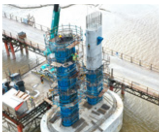
Prefabricated Pier 预制墩柱
