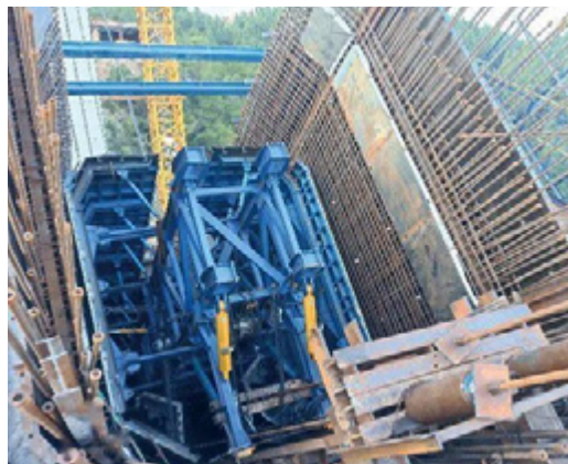
Cantilever Carriage for Arch Bridge 拱桥挂篮
