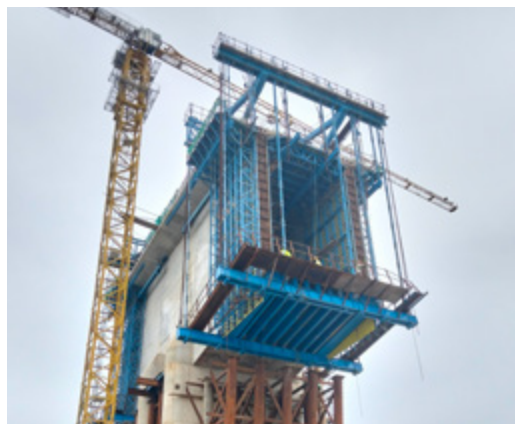
Balanced Cantilever Carriage 挂篮
