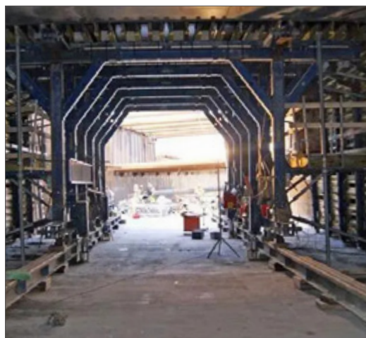
Timber Formwork Pipe GALLERY Tunnel Trolley 木模体系台车
