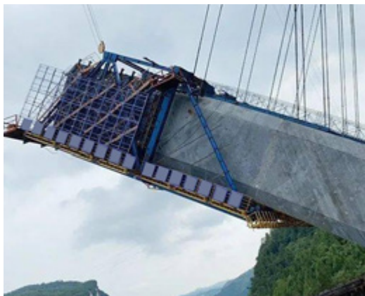
Cantilever Carriage for Arch Bridge 拱桥挂篮
