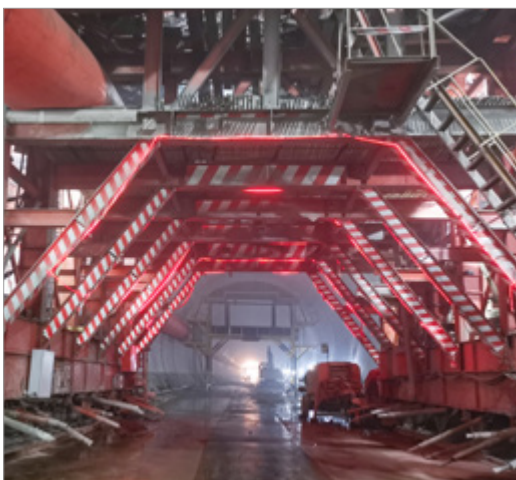
Steel Formwork Tunnel Trolley 钢模体系隧道台车
