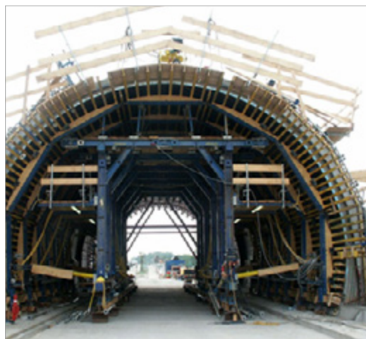
Timber Formwork Tunnel Trolley 木模体系隧道台车
