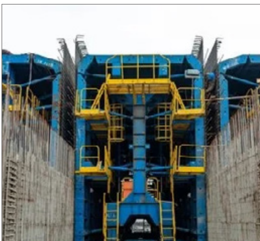
Steel Formwork Pipe GALLERY Tunnel Trolley 钢模体系管廊台车
